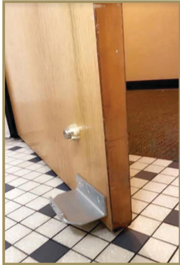
Work has been done to reduce common-touch surfaces in the house.
